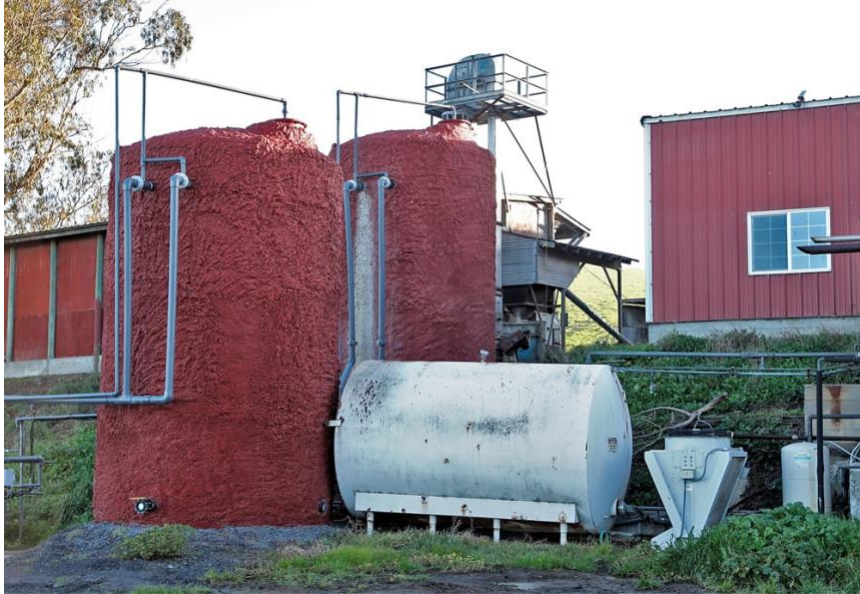
A methane digester stands on Straus Dairy Farm in Marshall, California. Scott Strazzante / The San Francisco Chronicle via Getty Images
